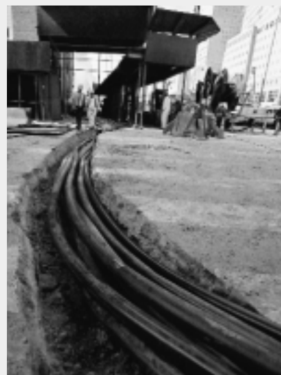
Figure 3 Temporary Cable Runs Bypassing WTC Areas
