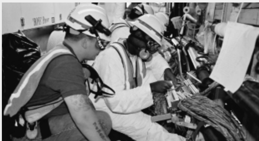
Figure 2 Verizon Technicians Repairing Cable at 140 West Street Facility Damaged by WTC Building #7 Collapse
